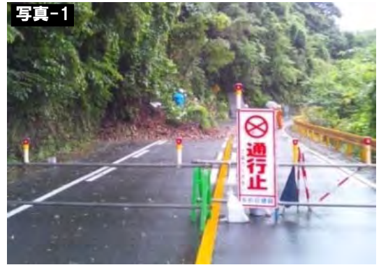
▲H25.9被災状況(長門市俵山)
